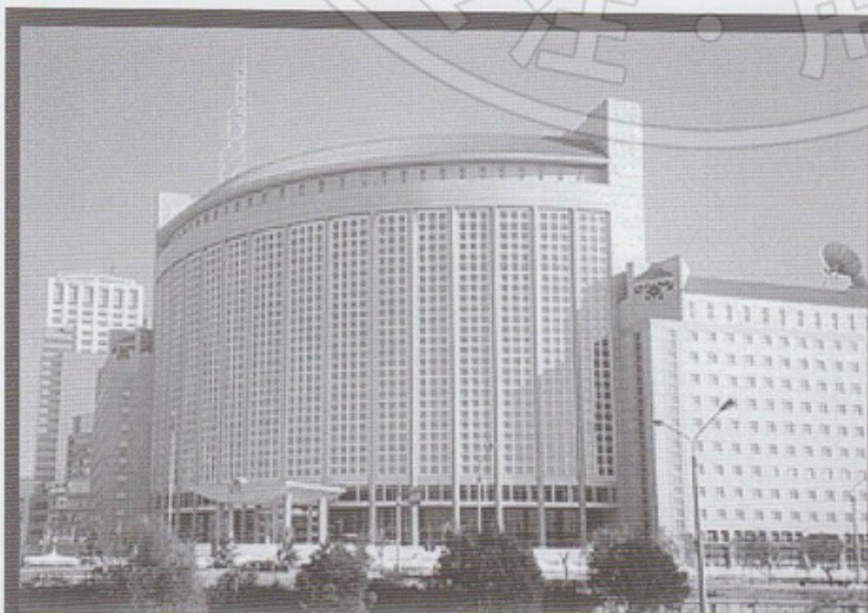
National Diplomatic Office Building (Beijing) 国家外交部办公大楼
